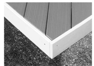
End-to-End or End-to-Trim = Gap according to estimated expansion table.
